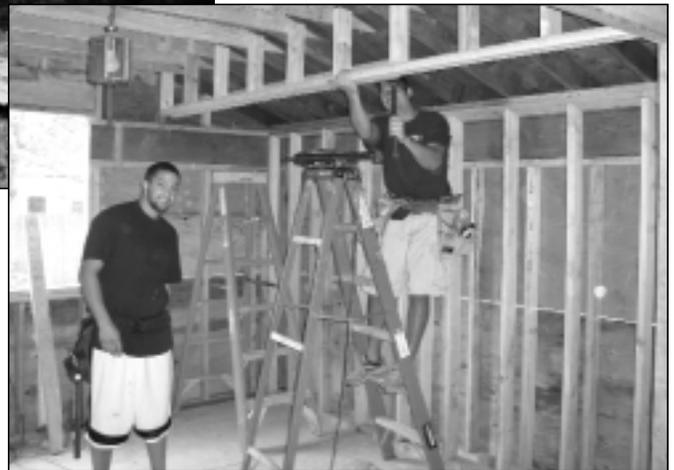
**Above: Joe Scelfo (on ladder) of Scelfo General Contracting and crew member work on the addition of the fully accessible kitchen. Other areas of renovation include equipping two bathrooms with ADA-compliant fixtures and grab bars, one with a roll-in shower; adjusting two bedrooms to allow for wider hall space; converting the garage into rooms for medication, storage and laundry; and building ramps for improved accessibility.**
